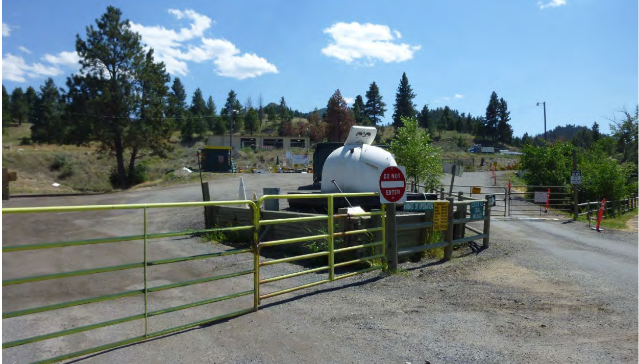
Montana City Container Site Entrance
