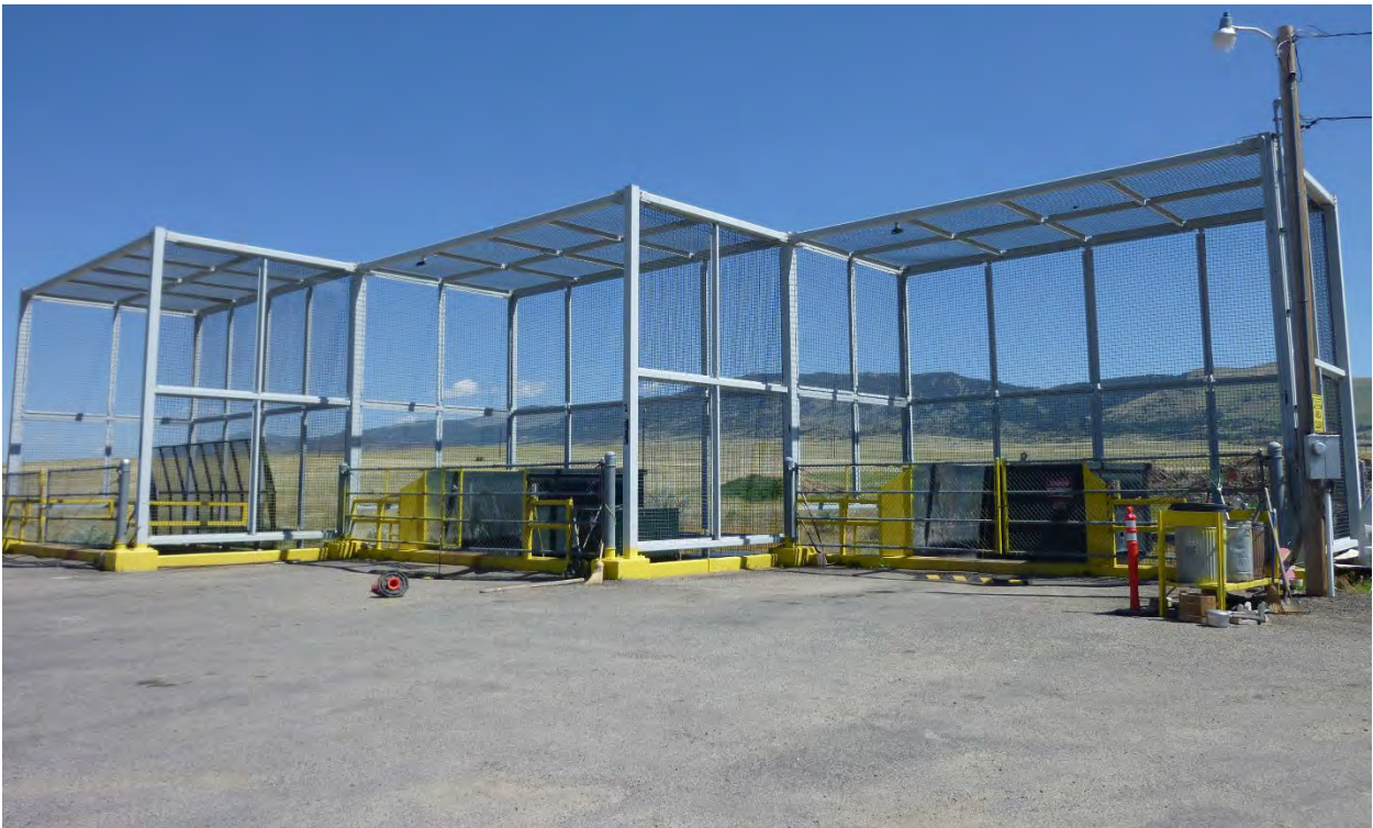
Whitehall Container Site
